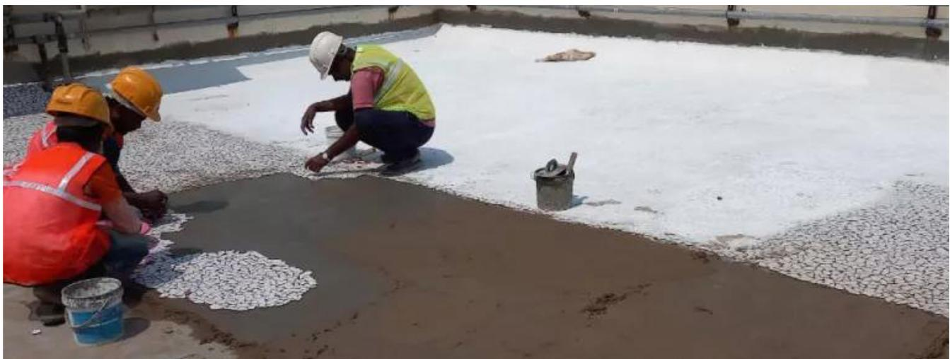
Figure 4: Mosaic Roof Installation in Kompally, Hyderabad, Telangana.
